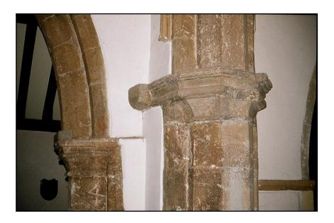
In medieval times there was a corbel on each side of the Chancel arch, to support the great Rood beam. The beam sometimes sat on the top of the screen, but some were placed slightly higher than the screen. Others could even be walked across. However, they all held a large Cross (or Rood) in the centre, with the figure of Christ nailed on it and the statues of St Mary and St John, one on either side.
